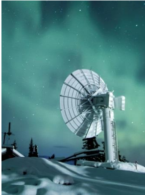
Ground Segment Infrastructure
