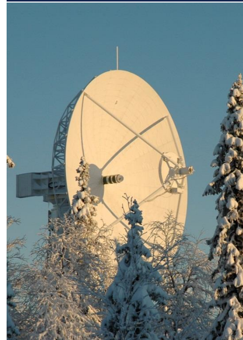
Satellite Ground Network
