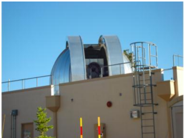
Figure 72: OCTL telescope will be modified with an optical flat to support links in the presence of more windy conditions.
